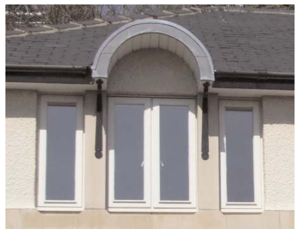
Arched window detailing in Thomas Hawksley Park.
