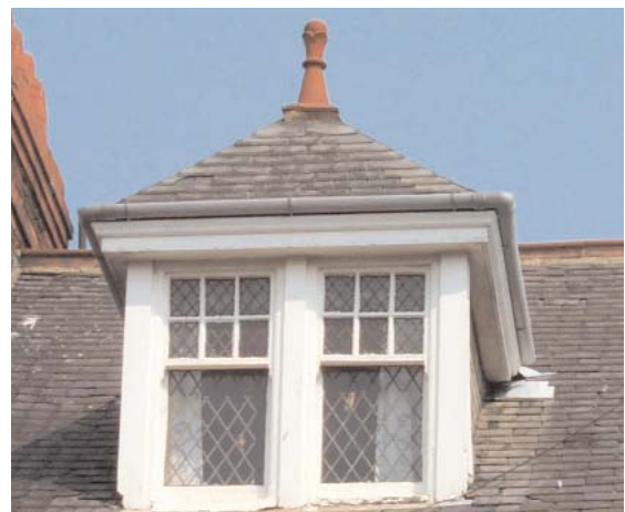
An original dormer feature with timber sliding sash windows, a welsh slate roof and a terracotta finial to the top, repeated along the terrace at Cedars Gardens
