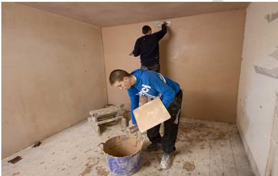
Figure 6: Plastering training course at Hylton Skills Campus
