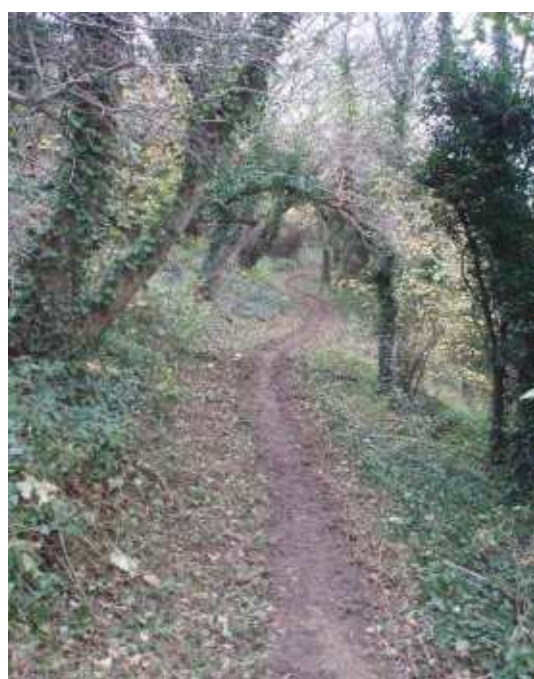
Footpath before clearance works carried out
