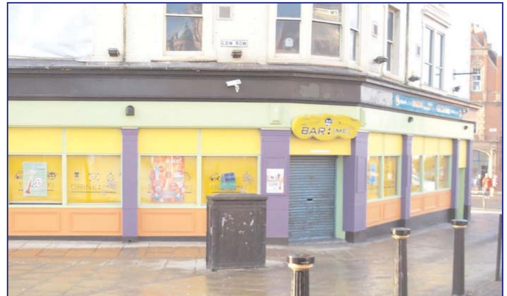
This pub frontage was formerly painted a traditional burgundy red which helped it to integrate with the building as a whole much more successfully than it does now.
