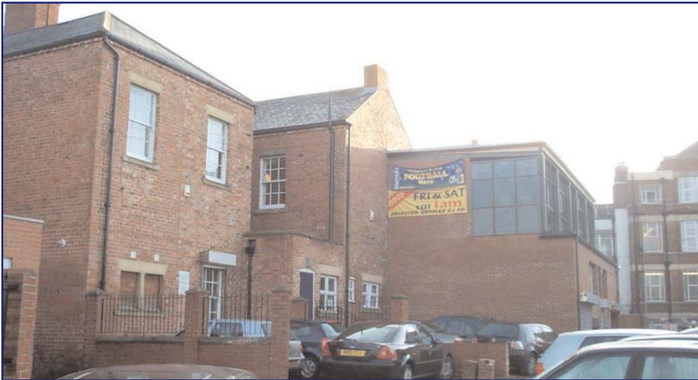
The rhythm and uniformity that originally characterised the rear of Green Terrace has been spoiled by the addition of the above extension.
