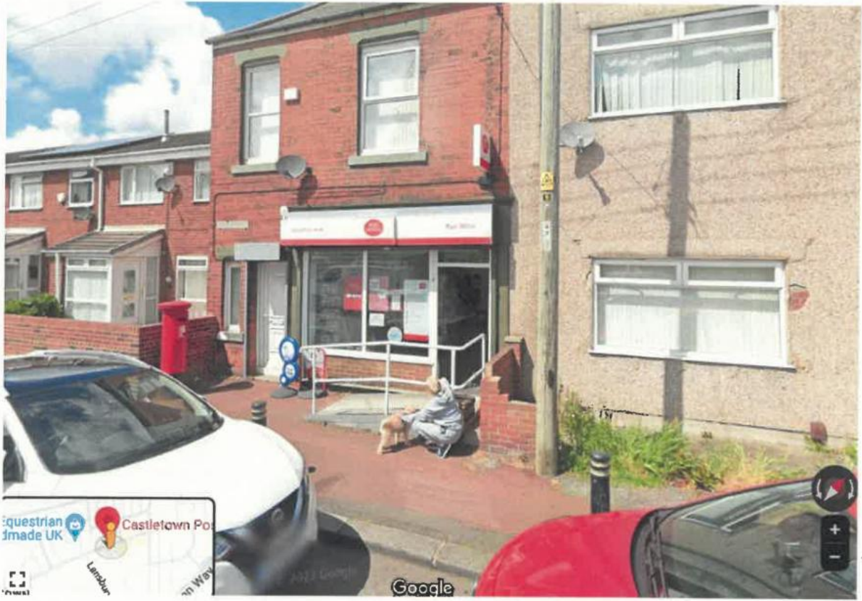
Figure 1 – Castletown Post Office
