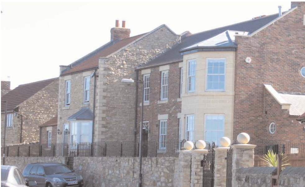
These recently built properties respect and reinforce the building line, form and materials of historic properties along North Street. The use of uPVC windows does however detract from the buildings and general street scene.
