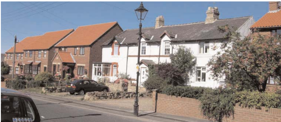
Picture showing adverse impact of insensitively designed new housing and boundary walls on the historic Front Street.
