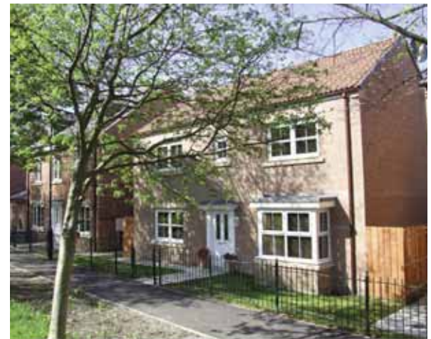
Station Road Penshaw
