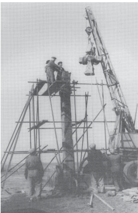
Bedes Cross under construction (1904)
