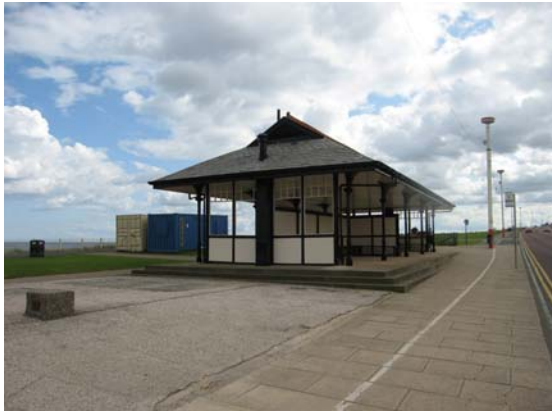
Seaburn upper promenade seating shelter
