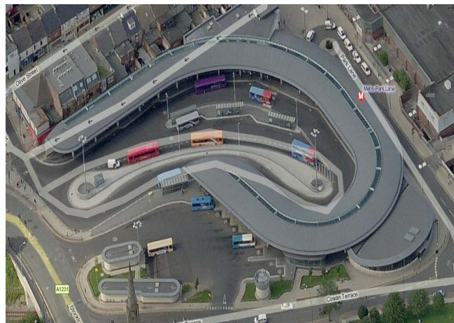
Park Lane Interchange
