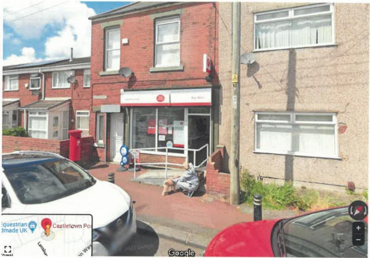
Figure 1 – Castletown Post Office
