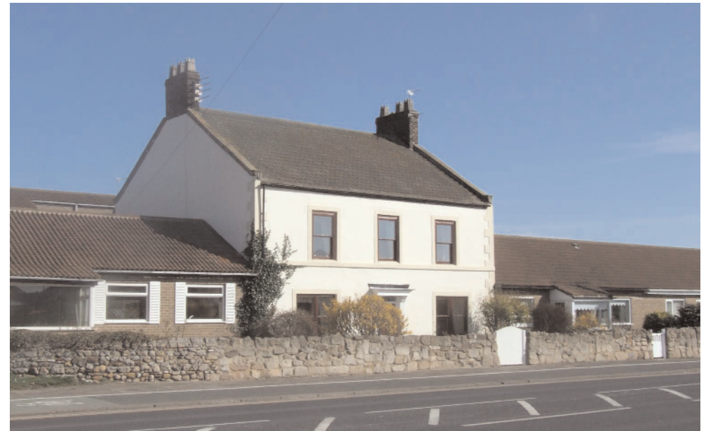
The bungalows built either side of South Bents Farmhouse detract considerably from the setting of this Listed Building. The materials used are particularly incongruous to the traditional character of the conservation area.
