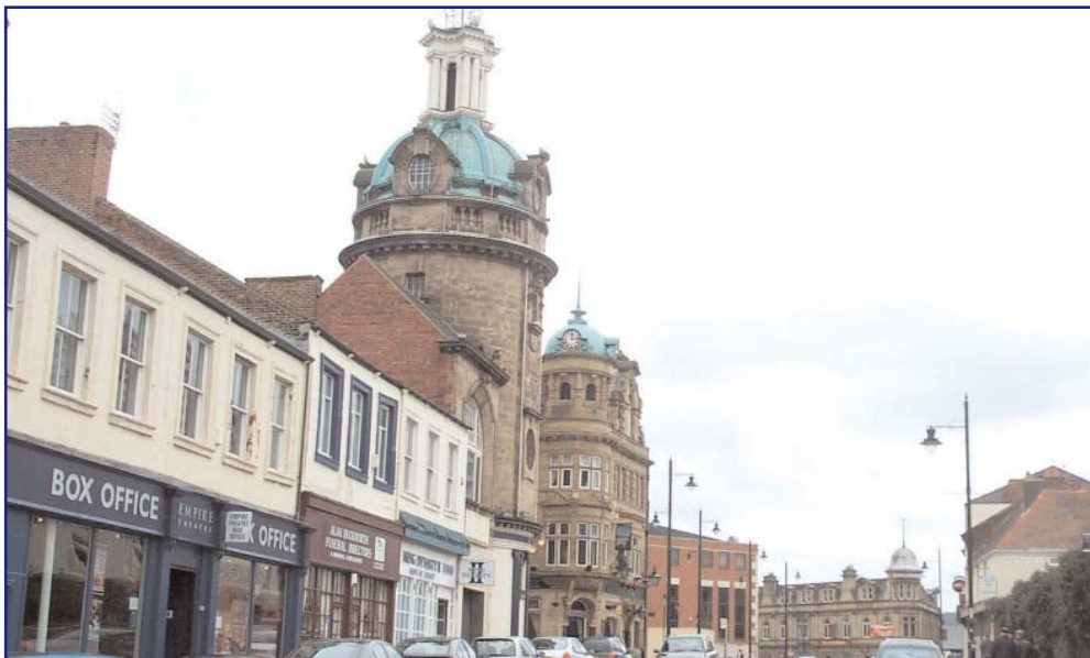
The variety building forms, styles and materials adds significantly to Bishopwearmouth's character.
