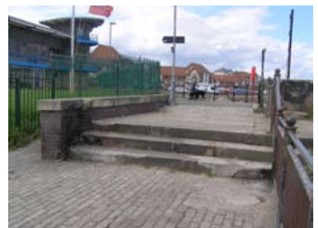
View from North Haven, facing north
