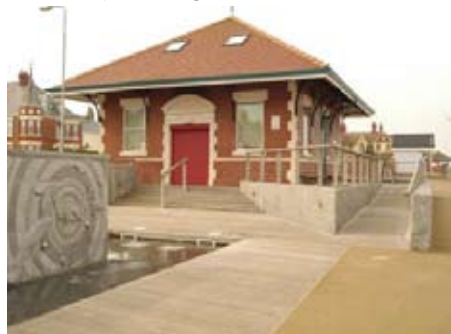
Covered depot building, Hornsea
