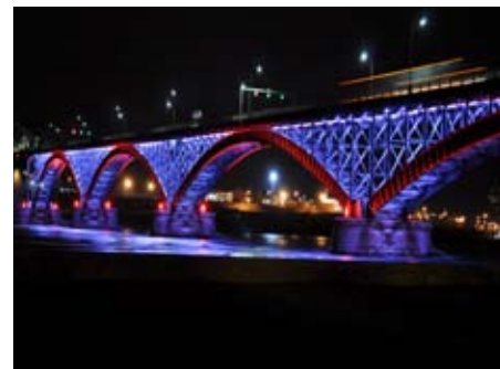
Example of an illuminated bridge
