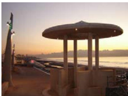
Promenade improvements at Cleveleys, Lancashire
