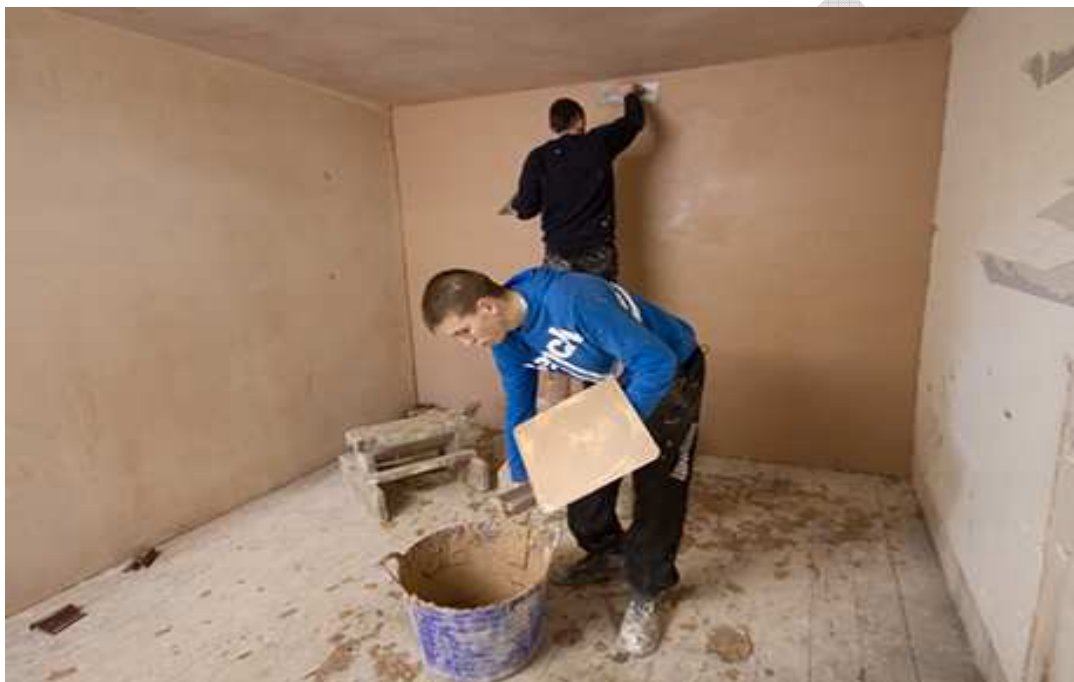
Figure 6: Plastering training course at Hylton Skills Campus
