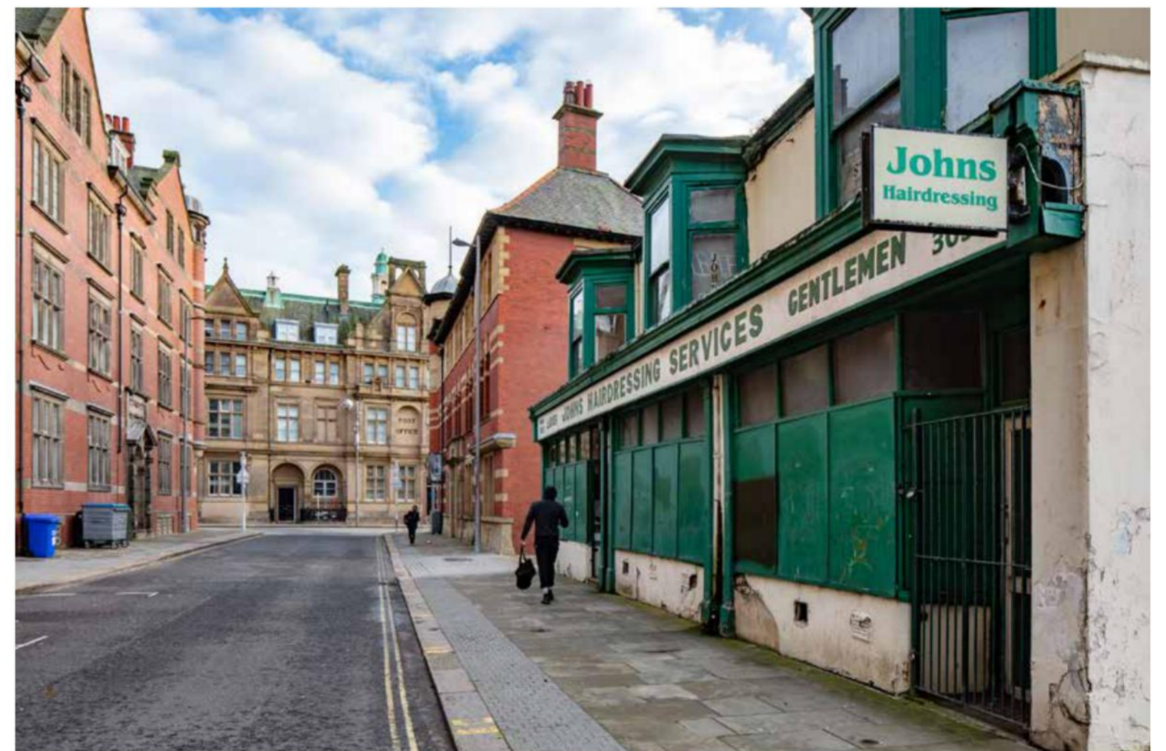
Boarded up shops and vacant properties create a sense of degradation and detract from the appearance of Sunnyside’s grand historic streets.
