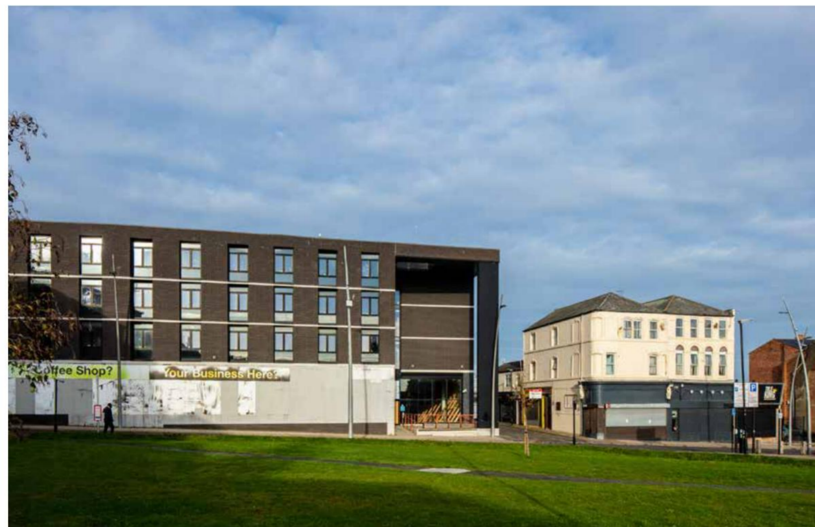
The former Travel Lodge is an area for congregation and anti-social behaviour
