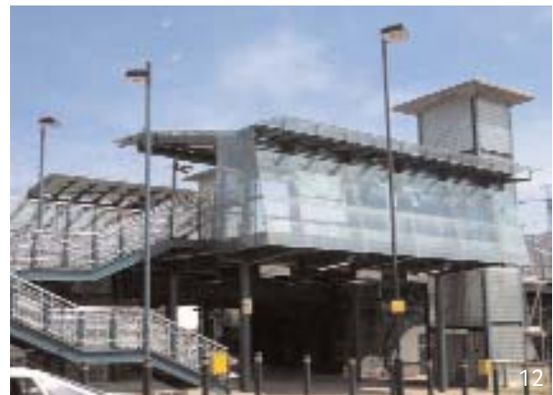
St Peter's Metro Station - Developers should consider how their scheme will link into the local public transport system.
