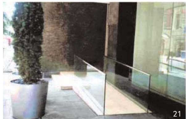
In this example the designer has integrated an access ramp into the overall design - thereby ensuring inclusive access.
