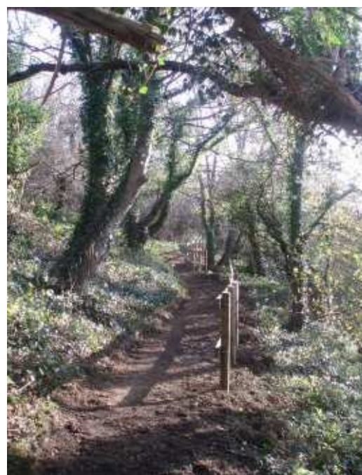
Footpath after clearance works carried out and edge protection installed
