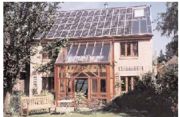
South facing Photovoltaics Oxford.
