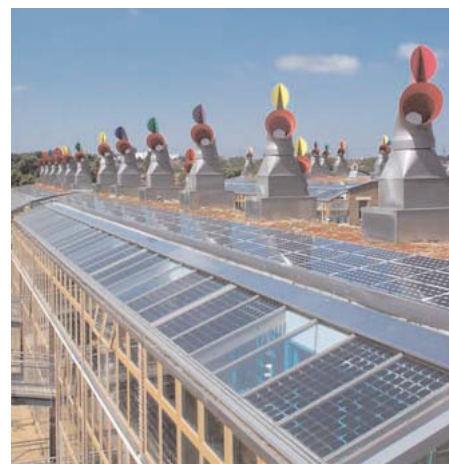
Photovoltaics in combination with a passive solar layout are used at BedZed, Surrey.
