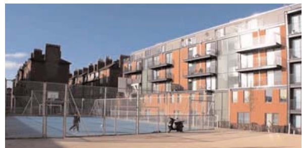
Beaufort Court, London. The high density site achieves significant open space between the blocks, unifying the new estate with the older adjacent site.
