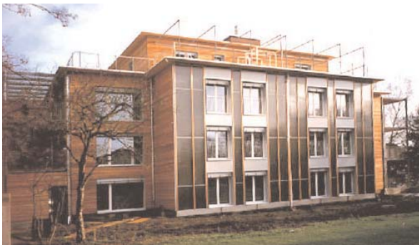
Trombe Wall, Rychenburg
