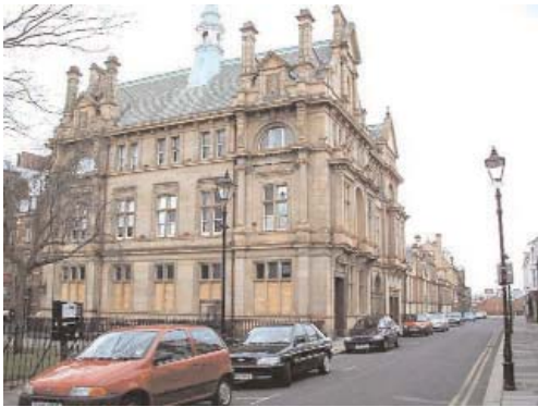
Building before conversion
