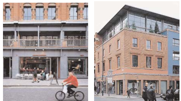
Smithfield Warehouse Conversion, Manchester. Mixed use block of apartments and offices with shops on the ground floor.
