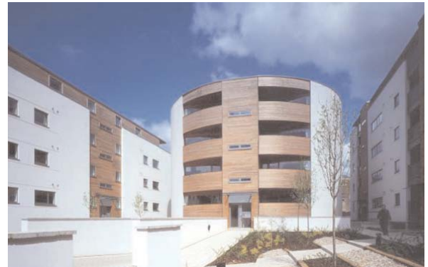
Century Court, Cheltenham. High quality amenity open space which is overlooked by adjoining properties.
