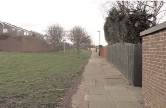
Houses backing onto public space detracts from the public realm and can compromise security and privacy
