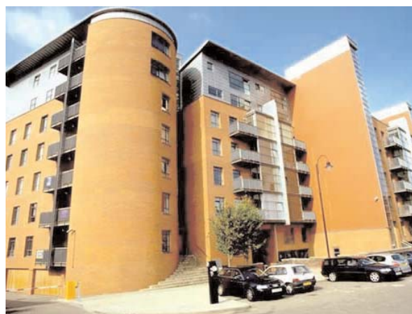
Deansgate Quay, Manchester
