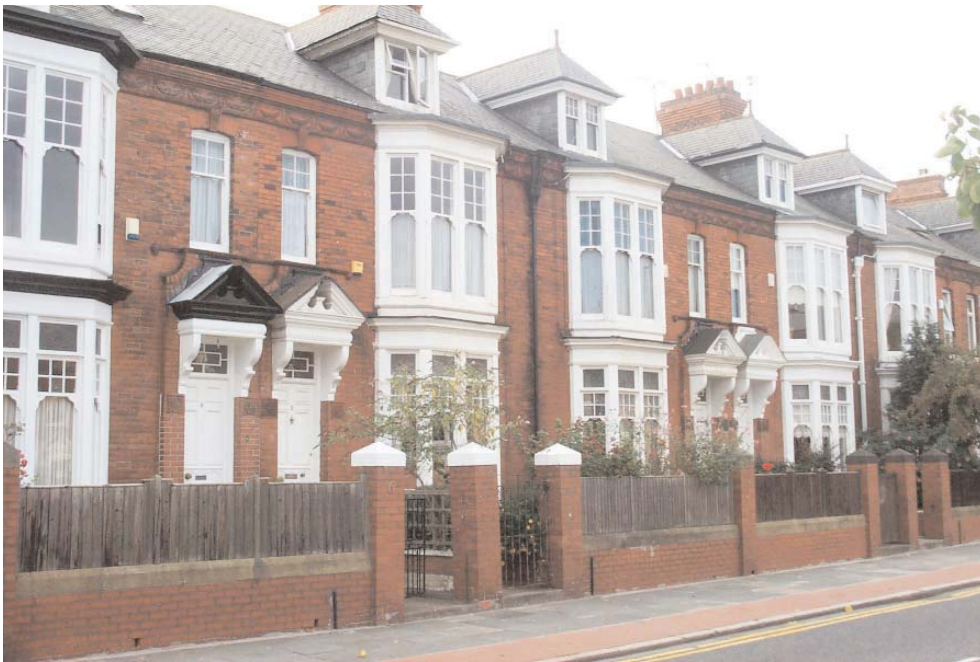
Repetition of impressive surviving timber features along Cedars Crescent
