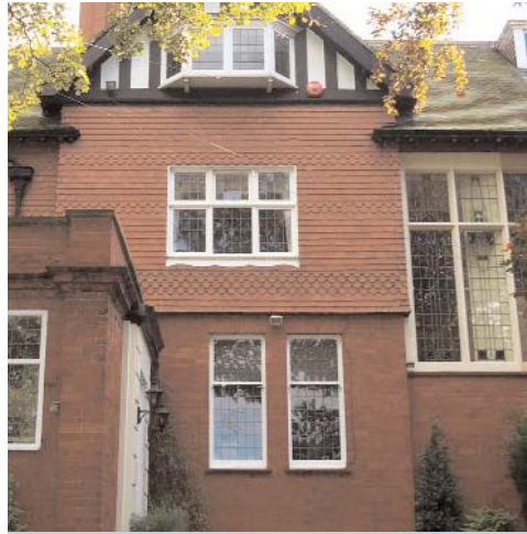
Terracotta tile hung front elevation
