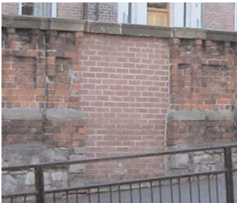
A former opening has been bricked up without regard to the original style, details or materials of the rest of the wall
