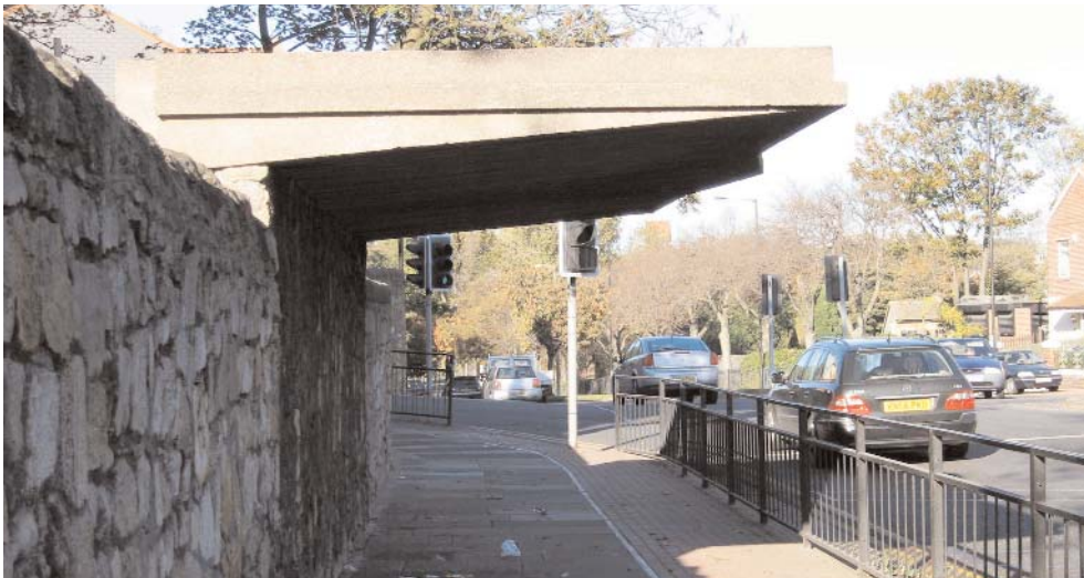
The disused bus shelter on Ryhope Road - to be retained or removed?
