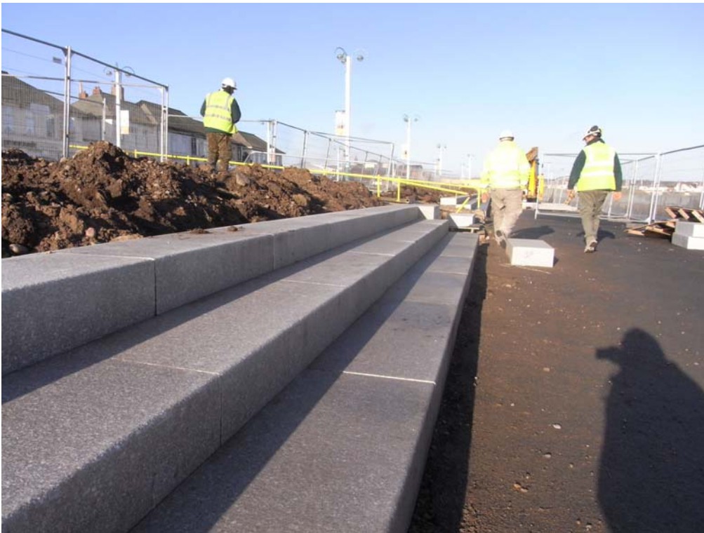
Photograph 2: New granite steps (January 2011)
