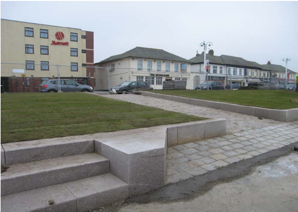
Photograph 3: Ramped access (February 2011)
