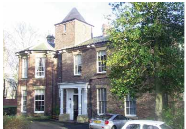
West Hendon House, Ashbrooke Conservation Area.
