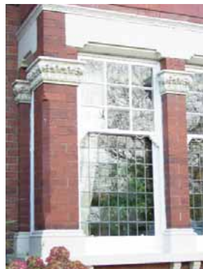
Rectangular shaped bays on Park Parade with decorative terracotta mouldings.
