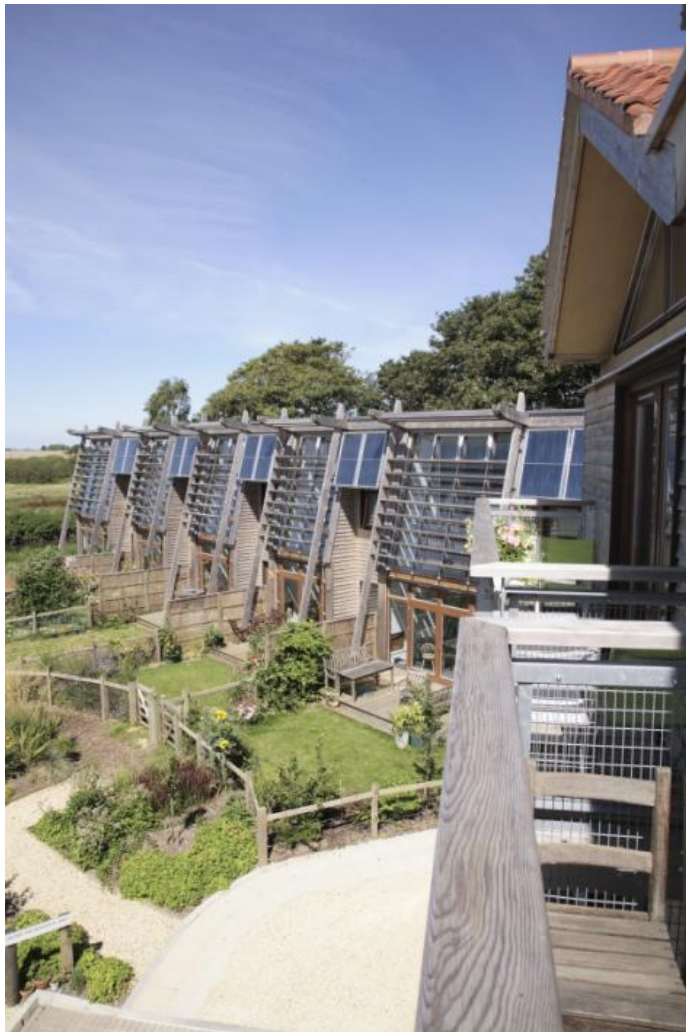
Ecos Homes Scheme, Great Bow Yard, Somerset demonstrating sustainable construction.
