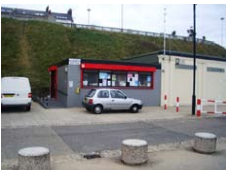
Poor quality buildings at Marine Walk
