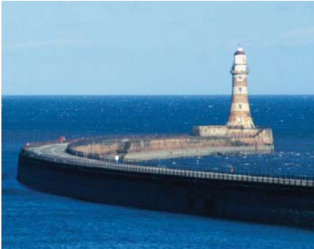
Roker pier and lighthouse
