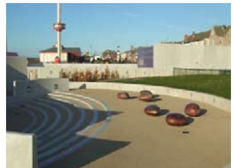
Resin bonded gravel
