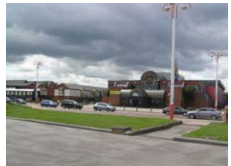
View from Ocean Park gateway, facing west
