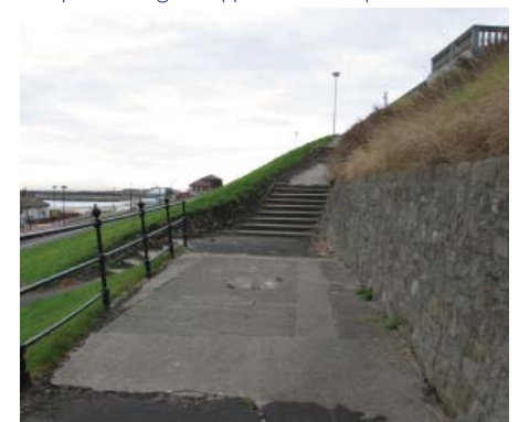
Footpath linking the upper and lower promenades
