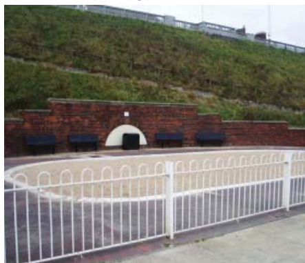
Unused former paddling pool
