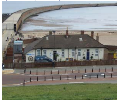
Lighthouse keepers' cottages
