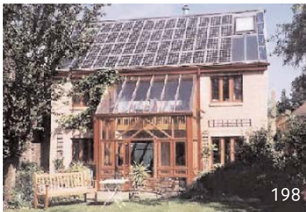
South facing Photovoltaics Oxford.
