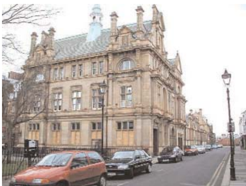
Building before conversion
