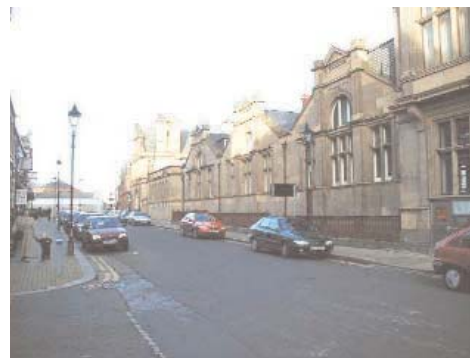
Building before conversion
