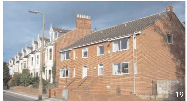
Poor response to context. New housing in the foreground fails to respond to the strong character and context of the existing terrace. The development does not respect the existing roofline, is devoid of detailing and neither harmonises or complements the original Victorian buildings.
