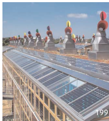
Photovoltaics in combination with a passive solar layout are used at BedZed, Surrey.
