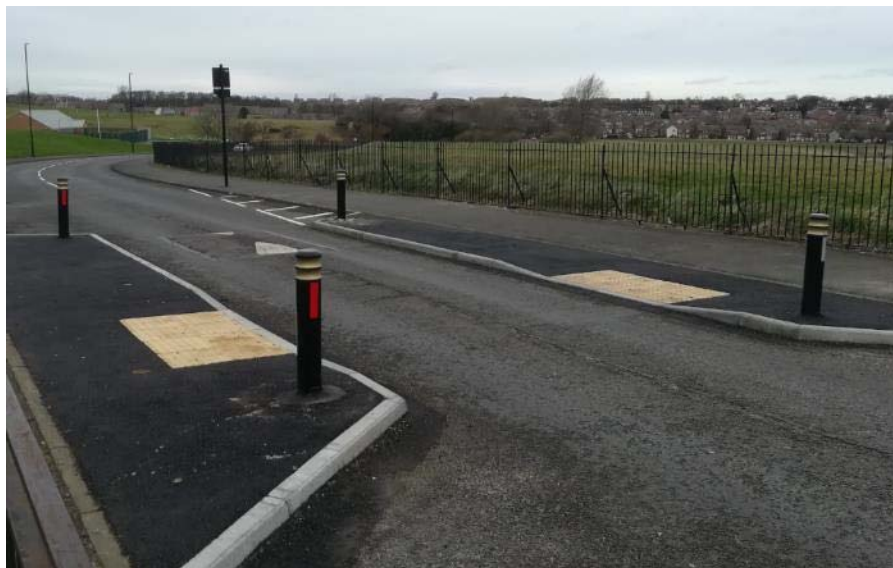
Traffic Calming Speed Reduction measures at Tay Road, Thorney Close
