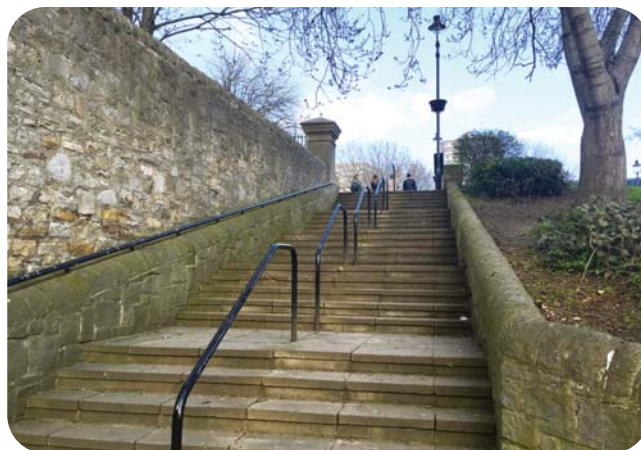
Figure 44: Photograph –Lack of natural surveillance at entrance steps into Town Park
