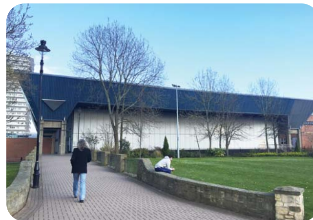
Figure 46: Photograph – Crowtree Leisure Centre presents inactive frontage onto Town Park
