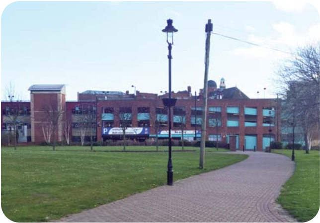
Figure 30: Photograph –Bridges Car Parking
