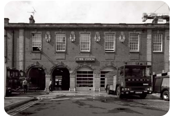
Figure 20: Photograph – Fire Station on Dun Cow Street
