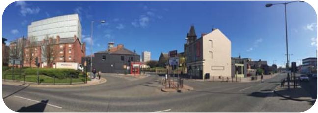
Figure 32: Photograph – Heavily Engineered junctions of St Michael's Way and High Street West Junction
