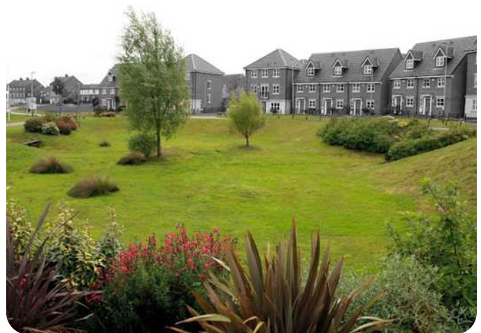
SUDS. Detention basin (susdrain)
